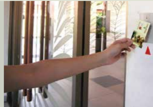
Tier 3: Security Access Card to the lift lobby via car park, and CCTV monitoring system for all entrances, exits and lift lobbies.
